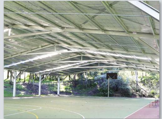
Safety and security under cover are also important. Ranbuild have removed the potentially dangerous diagonal wall braces and replaced them with lateral braces high up the columns and out of harm's way. Ranbuild COLAs also feature unique 'folded edge' column flashings to reduce the risk of contact with sharp metal edges.
